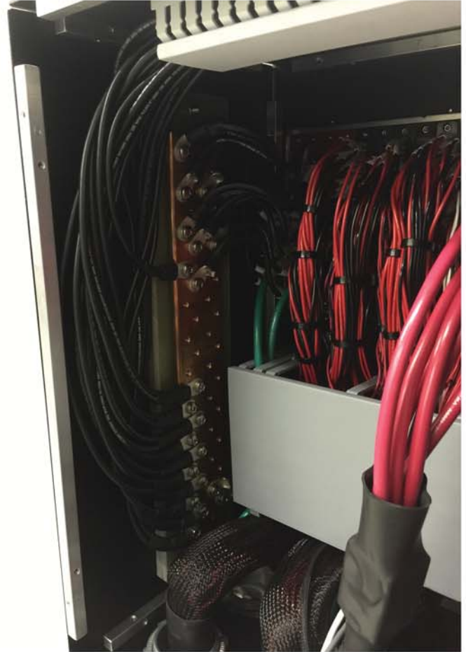
Inside ITA/Cable Harness with Bus Bars
